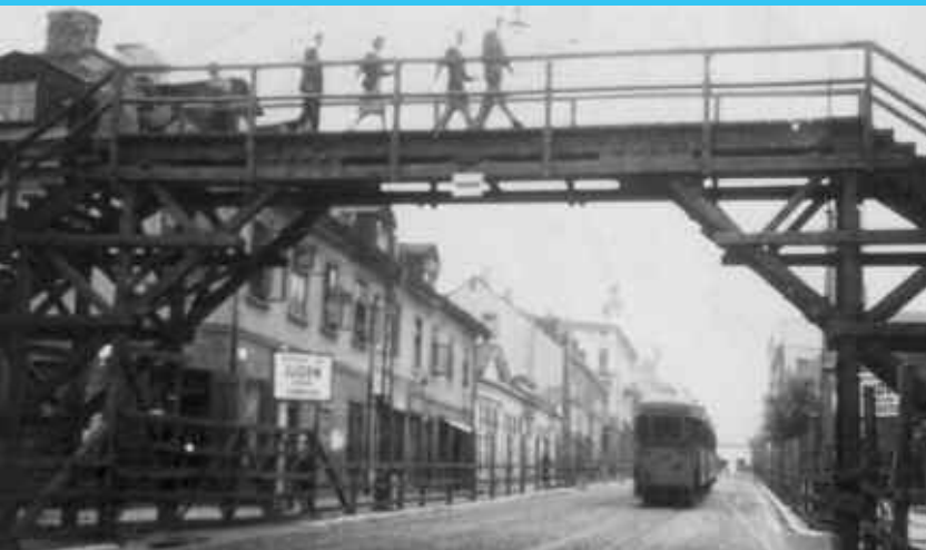
Footbridge over Zgierska St. near Podrzeczna St.
